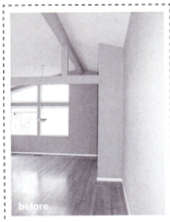
ABOVE: Two panels of an existing window and a partition wall in the original living room were removed to create more symmetry as well as space to accommodate the new kitchen and breakfast nook.
